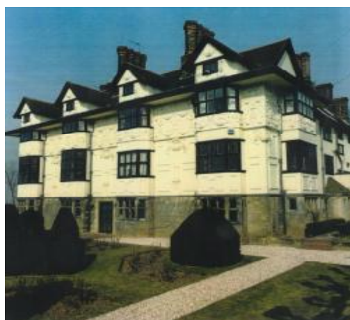
The Wood House
