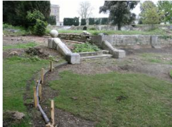
Garden restoration in progress
