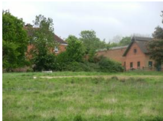
Little Copped Hall (left) with model farm building at Home Farm (right)
